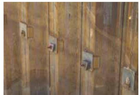
composition of well-granulated topsoil and fine-to-medium dense sand. In mid-winter, the general contractor, Scalamandre Construction, drove the sheet piles using a crawler crane with a fixed mast and an ABI variable moment. The driving settings were reduced to minimize vibration and noise to the surrounding neighborhood.
